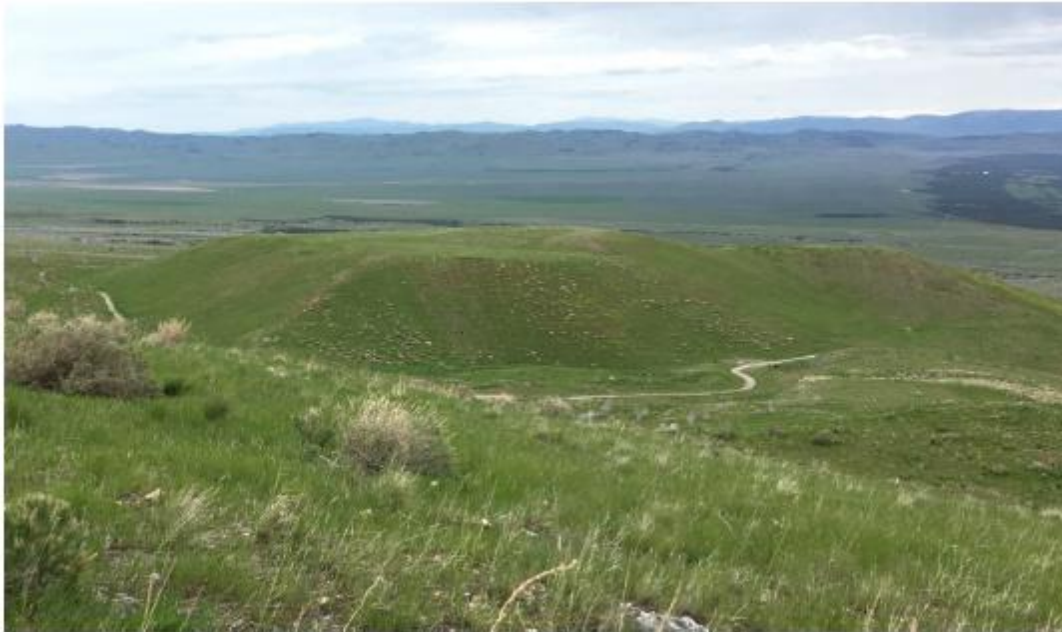
Figure 1 View of the Reclaimed Black Pine Mine Heap-Leach Pad, Looking East
